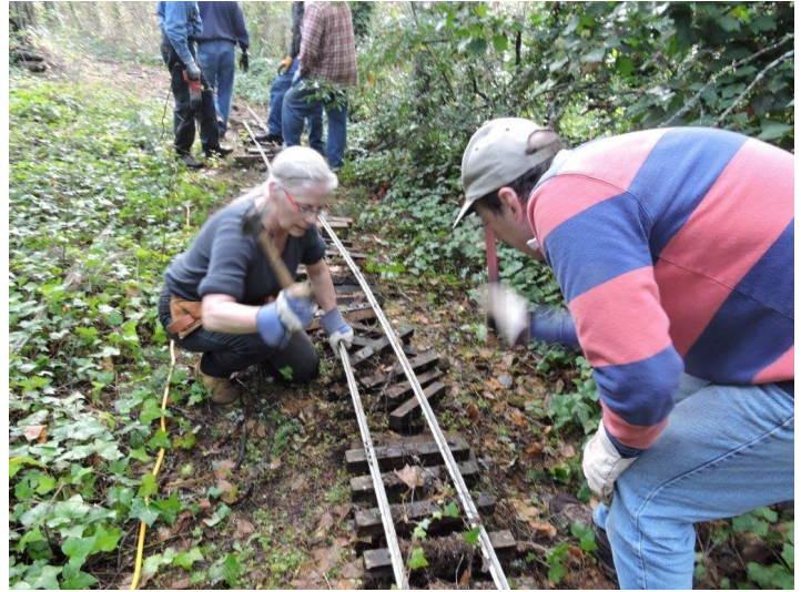
Pete and Dawn, hammers in hand, synchronize blows to the tie which usually popped off in one blow. In the background Terry with the Sawzall prepares to cut through a joiner, while Alex lifts track sections to make our jobs easier.
